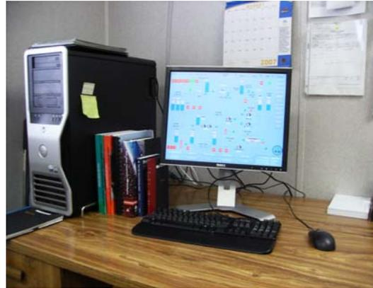
This is the mainframe computer for the telemetry system. This computer has dedicated power and communication lines to ensure seamless operations.
