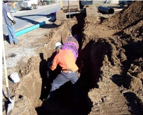
This crew is installing some ductile iron pipe that is wrapped in a purple plastic covering to indicate that the pipeline contains recycled water.
