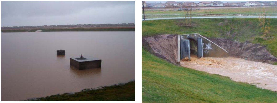
Figure 4-15 Stormwater in Eighth St. Basin (left) and discharging into Cherry Avenue Basin (right)
