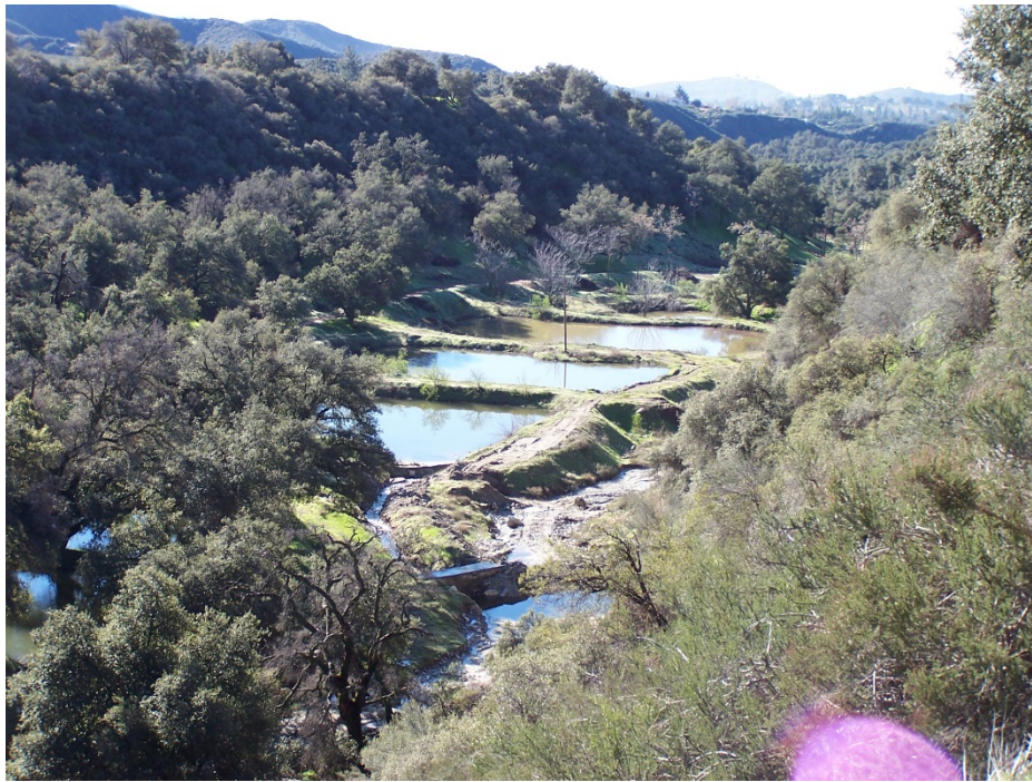
Figure 6-7 Percolation Ponds in Upper Edgar Canyon
