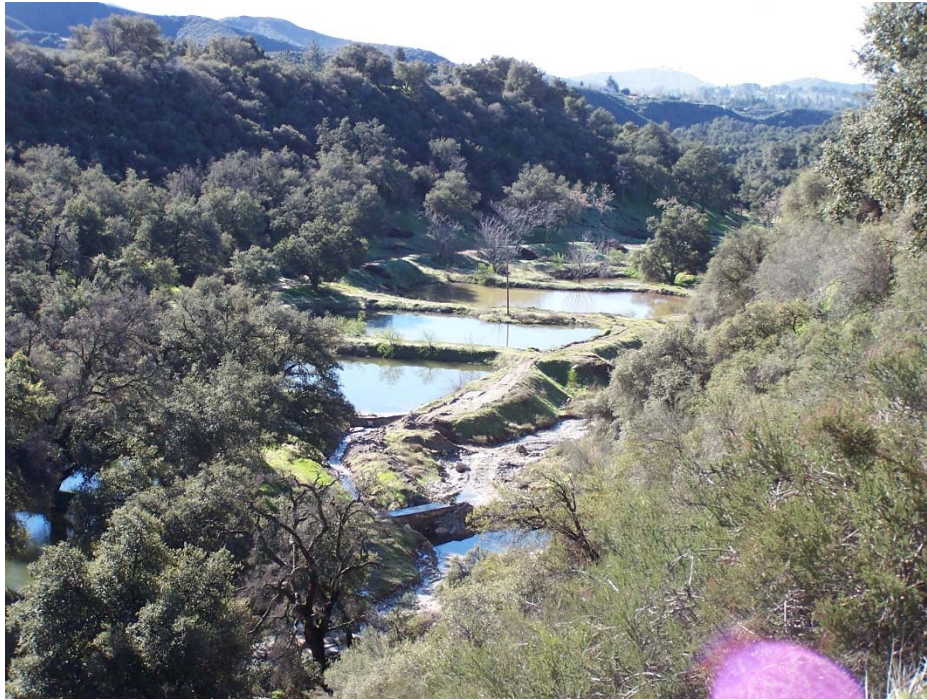
Figure 6-7 Percolation Ponds in Upper Edgar Canyon
