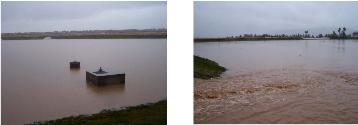
Figure 6-10 Runoff Collected in Sundance Detention Basin
