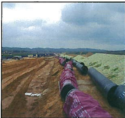
Purple recycled-water transmission mains ready for installation.
