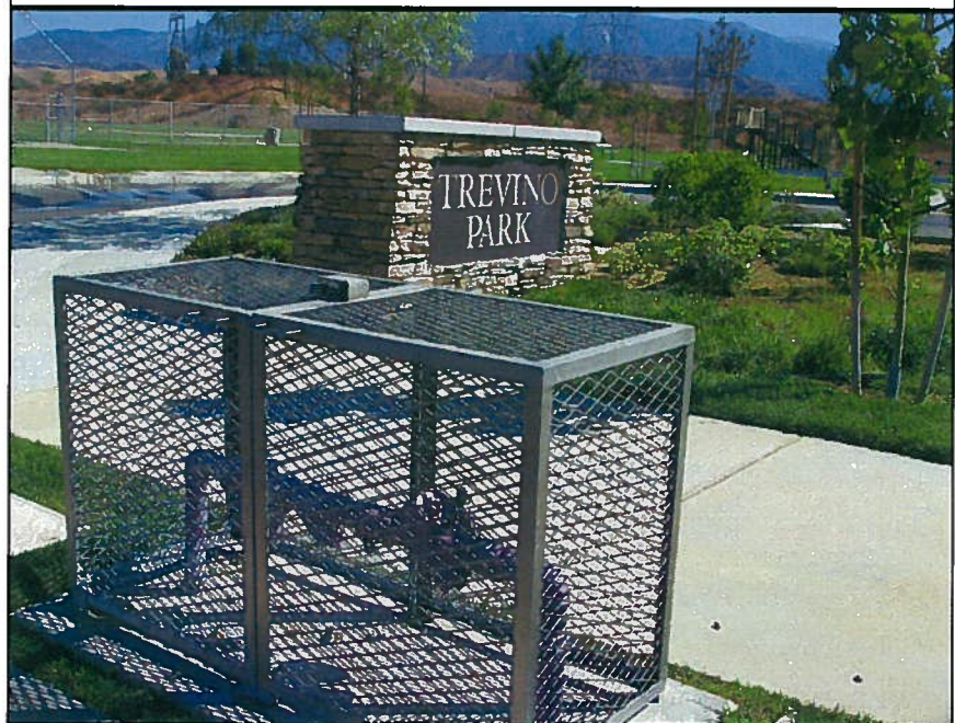
A Recycled Water System purple painted backflow device at Trevino Park at Fairway Canyon.
