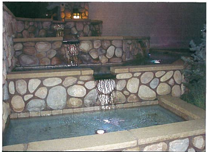
The BCVWD Headquarters fountain will use recycled water when the Recycled Water System is completed in 2010.
