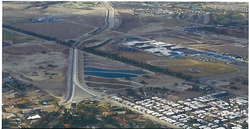
An aerial view, looking southwest, of the BCVWD Recharge and Recreation Facility with two recharge basins in operation.
