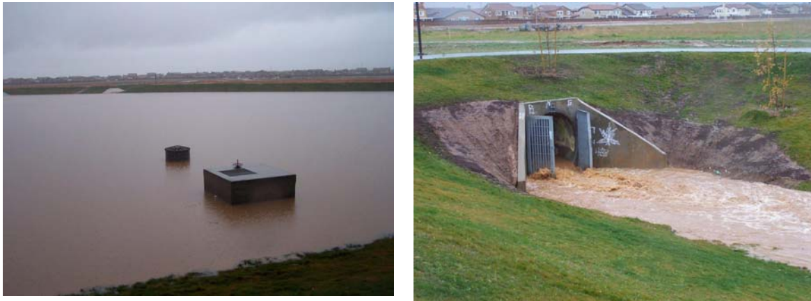
Figure 4-15 Stormwater in Eighth St. Basin (left) and discharging into Cherry Avenue Basin
