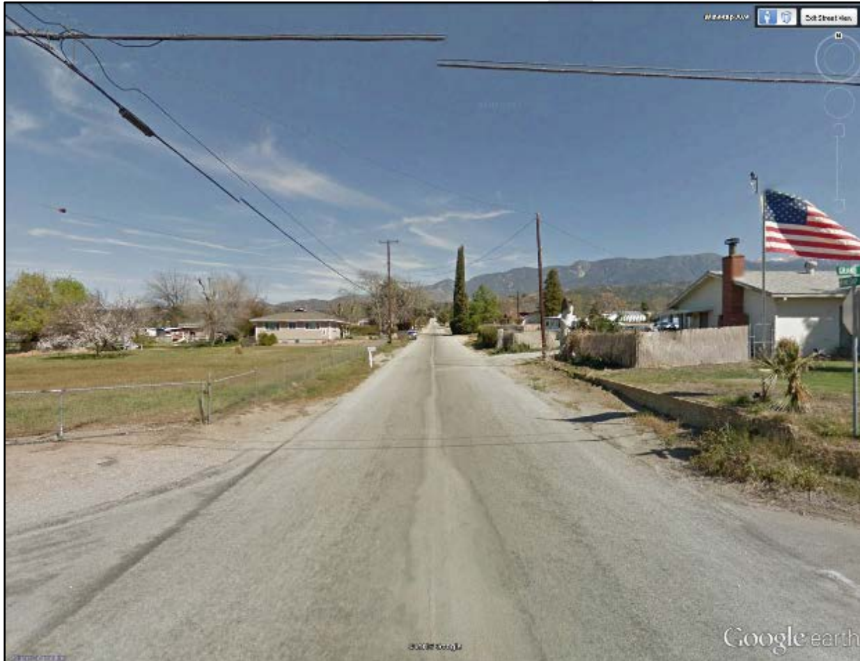
Figure 5: Winesap Avenue (at Grand Avenue intersection looking north) showing typical street with inverted cross section
