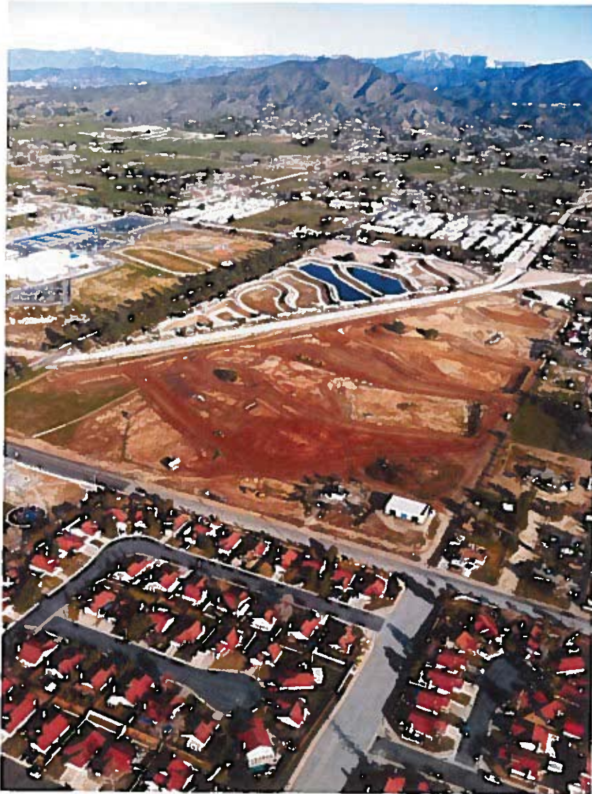
Noble Creek Recharge Facility
