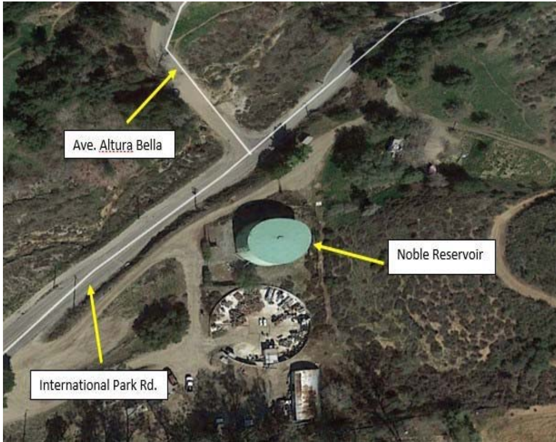
FIGURE 4 NOBLE RESERVOIR LOCATION
