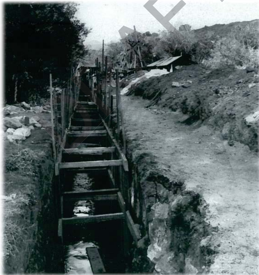
When well No. 2 was sunk north of Beaumont, it produced an adequate supply of water to the town, and a canal flume was built to bring it to Beaumont. The complexity of such an undertaking involved shoring up the canal wall, as can be seen in this photograph. (Courtesy of SGPHS.)
