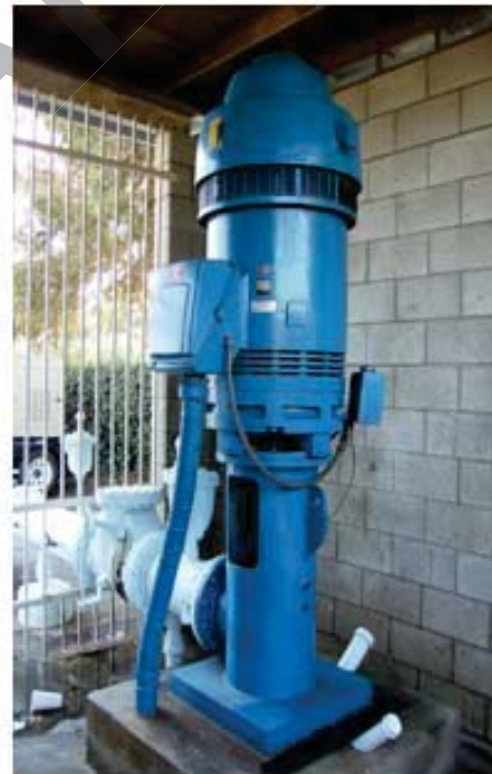
This is Well 1 today updated with a more efficient and modern pump.
