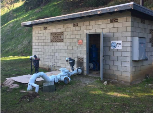
Well 4A Building
