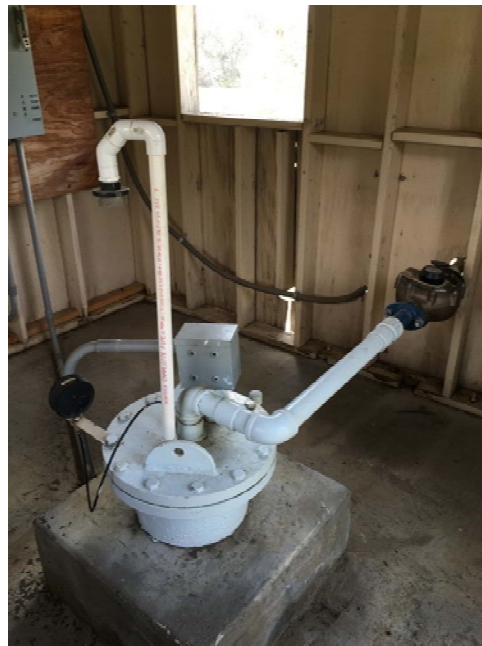
Well 18 Discharge Elbow and Piping
