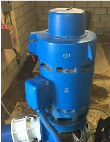
Well 4A Motor
