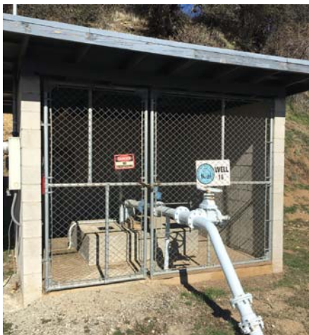
Well 10 Building Front View
