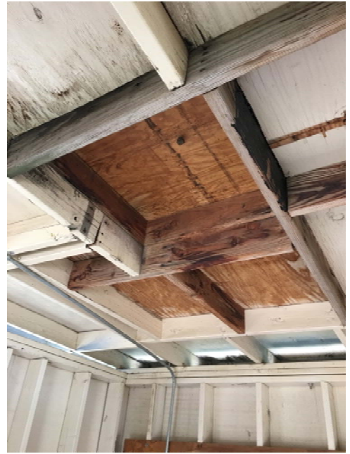
Well 18 Roof Hatch
