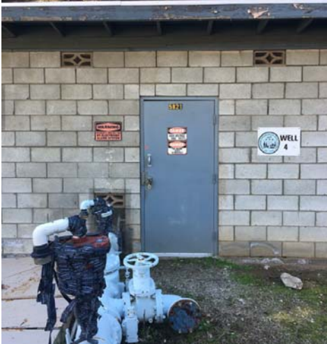
Well 4A Building Front View
