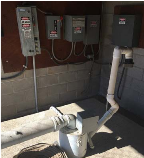
Well 10 Discharge Elbow and Piping
