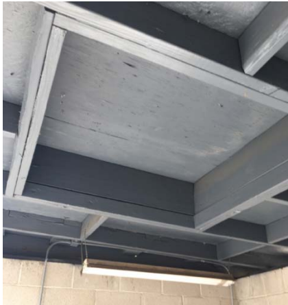
Well 10 Roof Hatch
