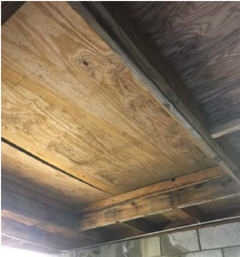
Well 4A Roof Hatch
