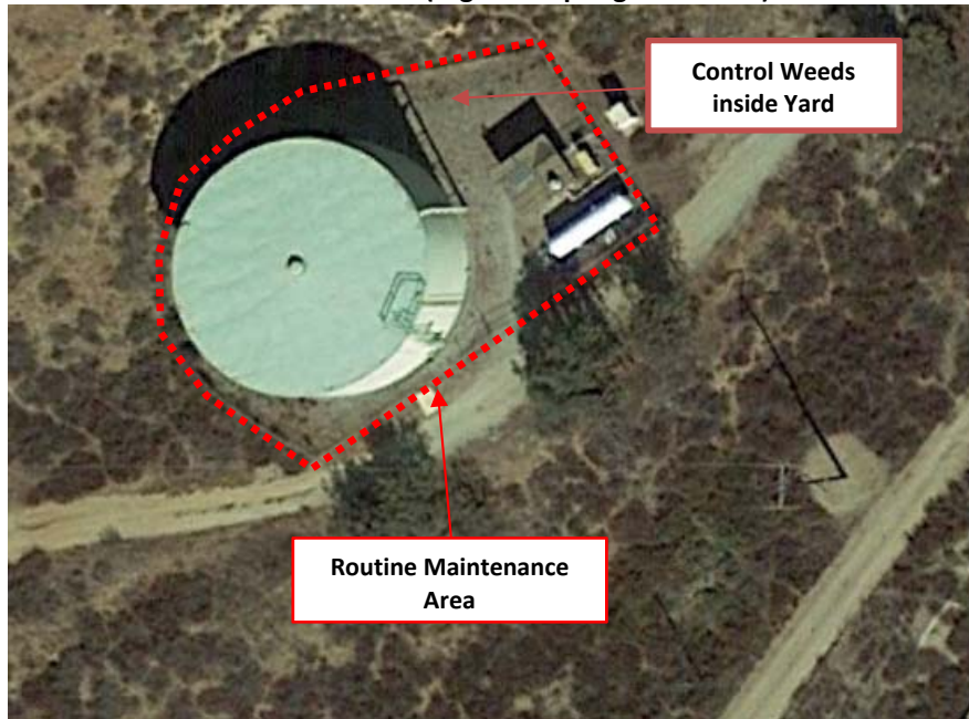
Figure 14 Site 14 – 3040 Pressure Zone (Highland Springs Reservoir)
