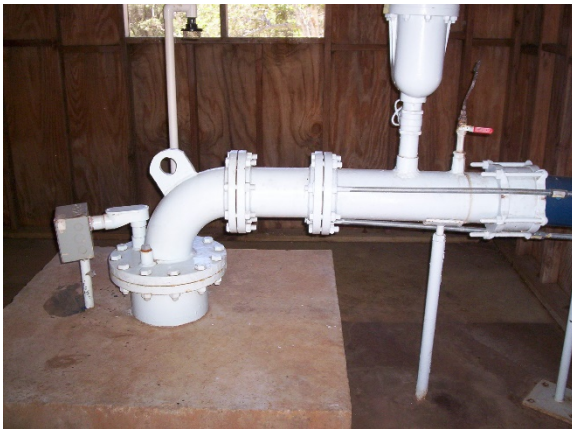
Well 14 Discharge Elbow and Piping
