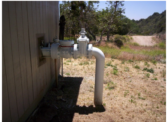
Well 14 Exterior Discharge Piping
