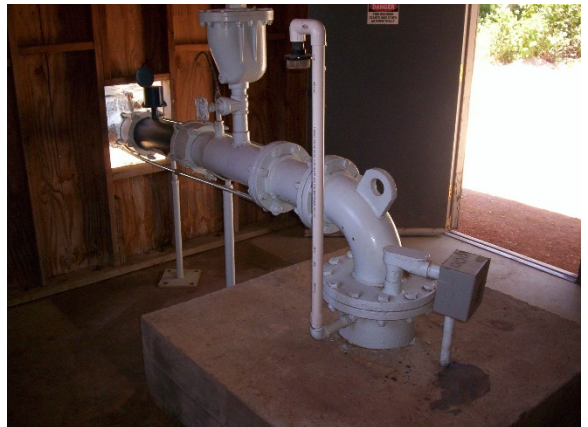
Well 14 Discharge Elbow and Piping
