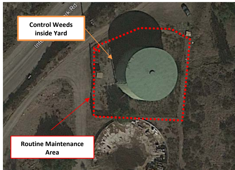
Figure 13 Site 13 – 3040 Pressure Zone Reservoir (Noble Tank)
