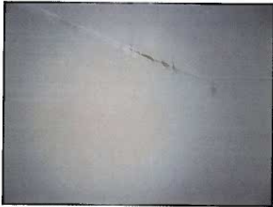
(#19) Wall Horizontal Weld Seam
