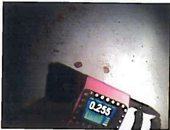
(#38) UT Readings Floor Quadrant 2
