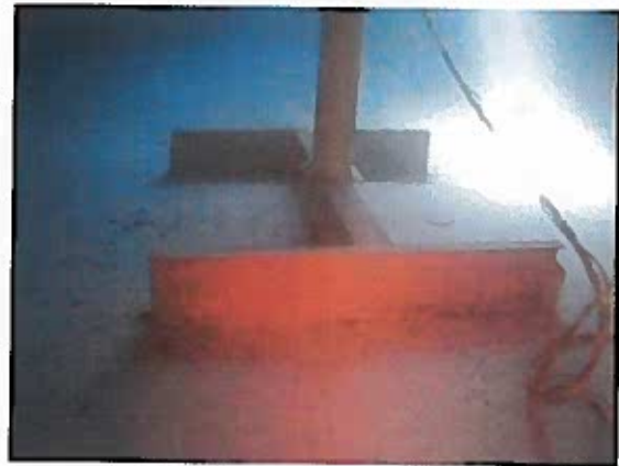
(#29) Center Column Base
