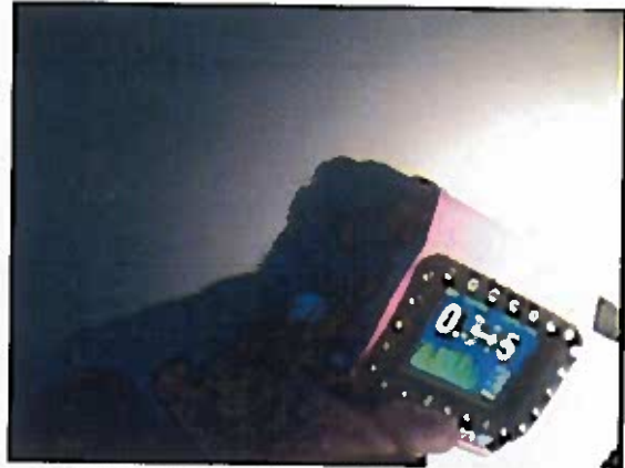
(#40) UT Readings Wall Quadrant 1
