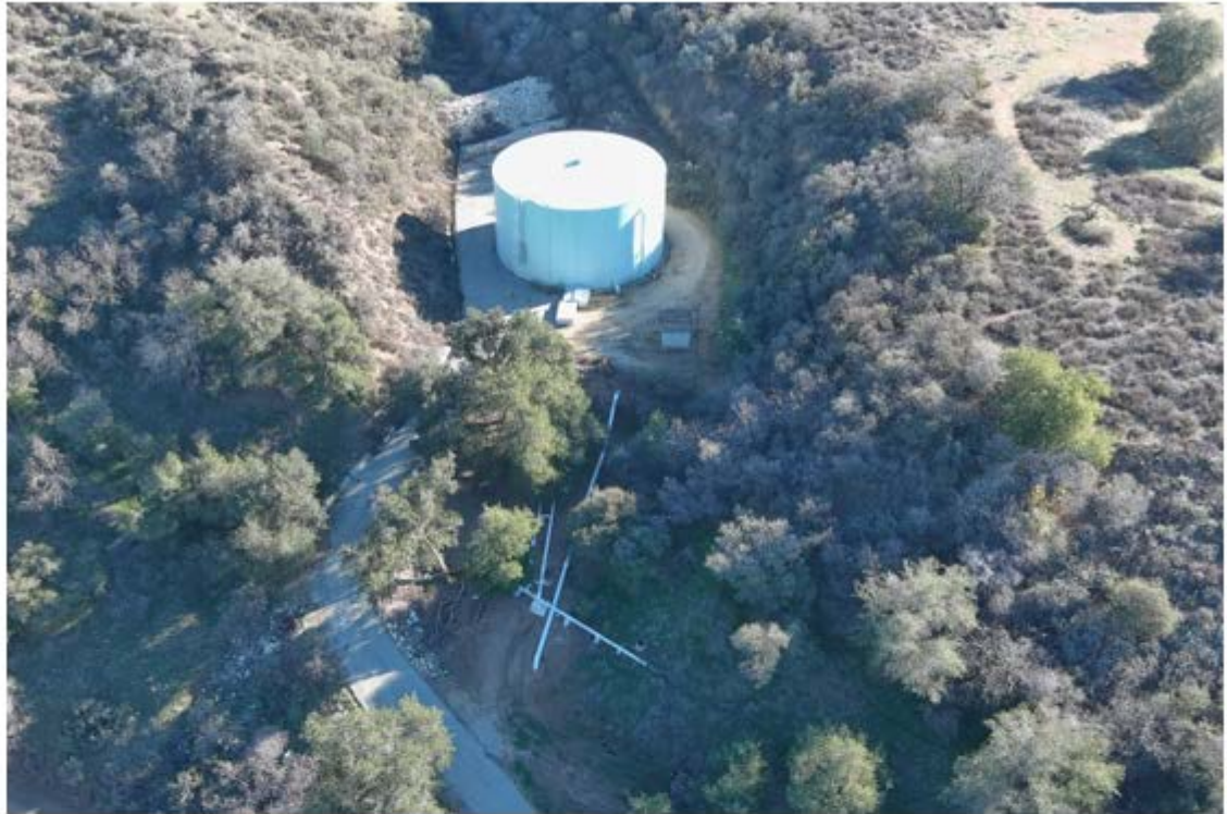
FIGURE 4 LOWER EDGAR TANK
