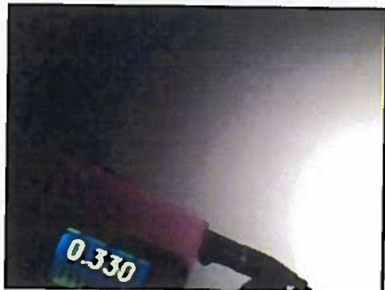
(#41) UT Readings Wall Quadrant 4
