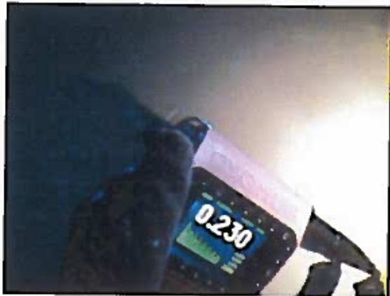
(#39) UT Readings Wall Course 2 Quadrant 4
