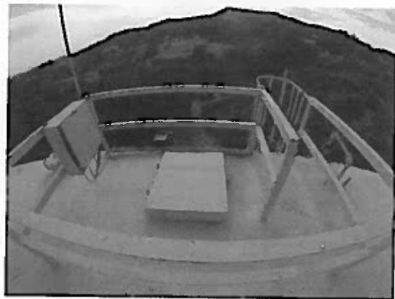
(#11) Roof Access Guardrail
