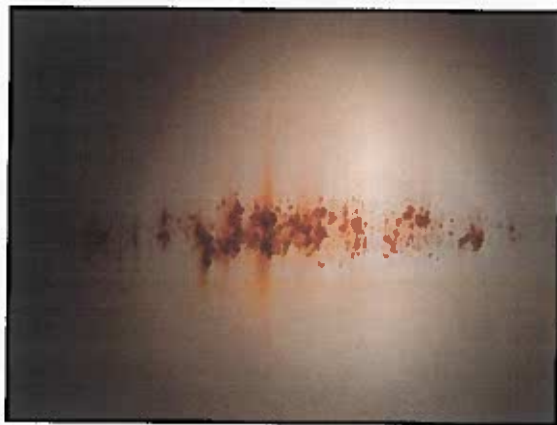
(#20) Wall Rust Nodules
