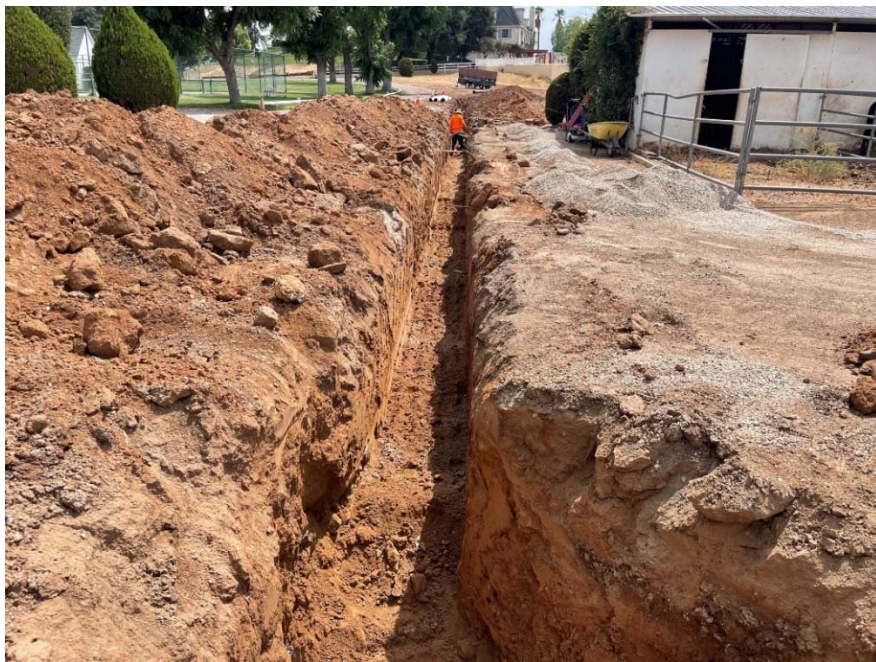
Figure 5: Open Trench of Pipeline 1
