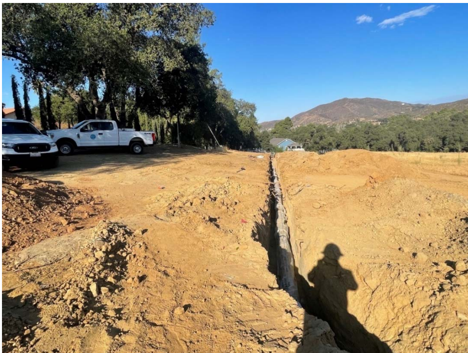
Figure 3: Pipeline 1 within Trench
