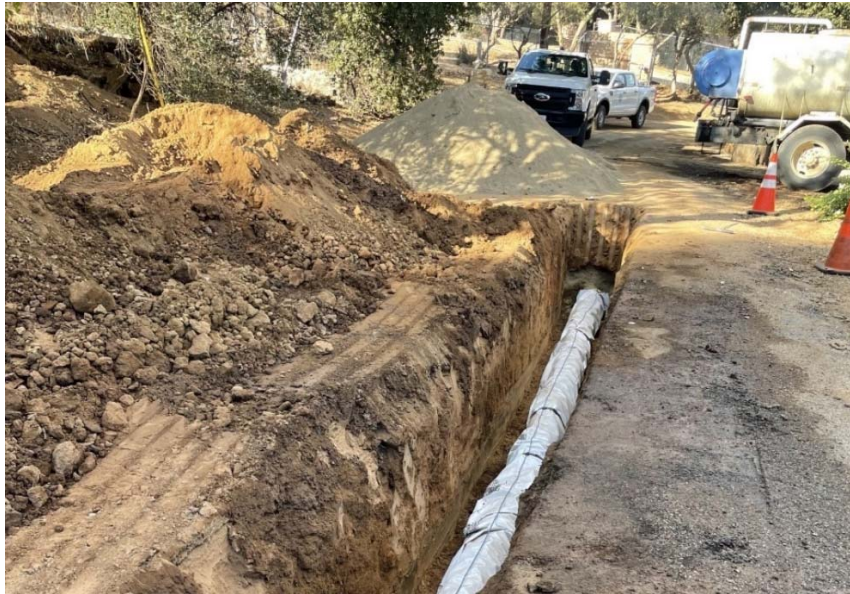
Figure 1: Polyethylene Wrapped Pipeline within Avenida Altejo Bella
