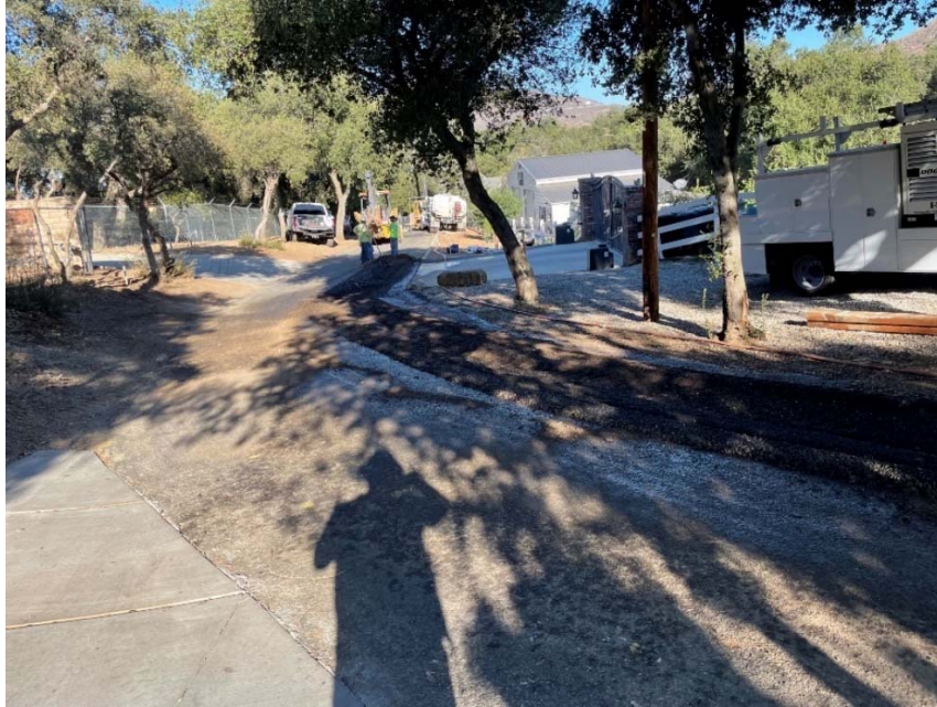
Figure 2: Temporary Trench (Pavement) Repair within Avenida Altejo Bella
